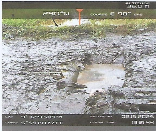
Fig 1. Incident point after exposing the pileline
