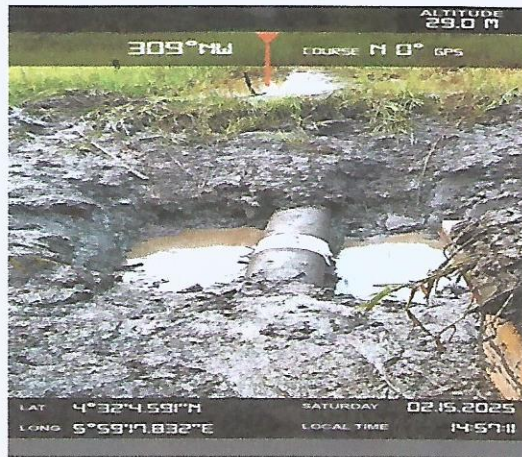
Fig 2. Incident point after repairs
